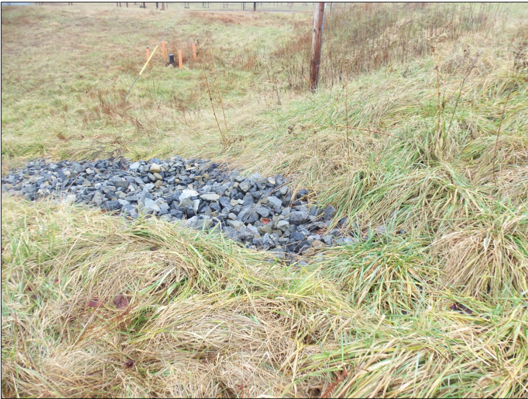
View of SWMU 40 Swale
