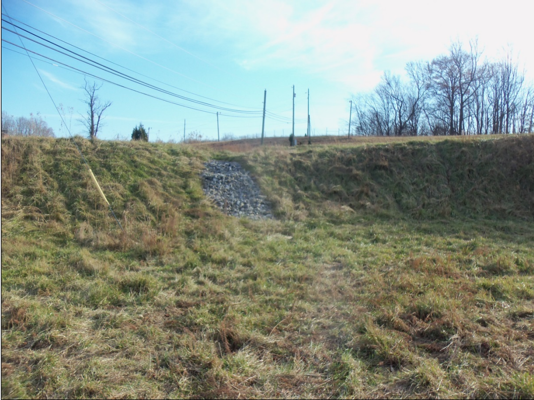
View to the North of SWMU 40
