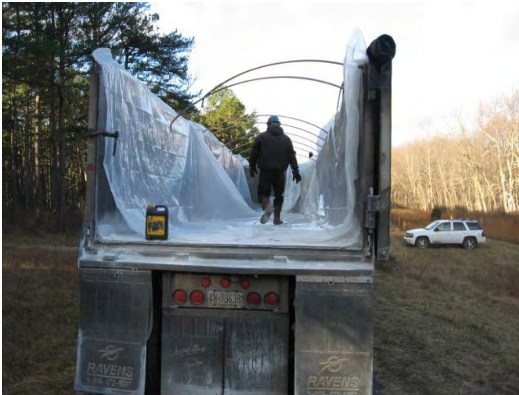
Photo 3 – View of plastic liner being installed in dump trailer prior to loading.
