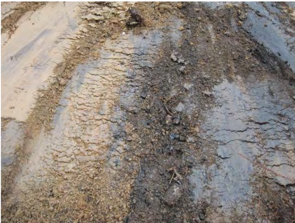
Photo 4 – Debris/ash from historic burning operations encountered during excavation activities.
