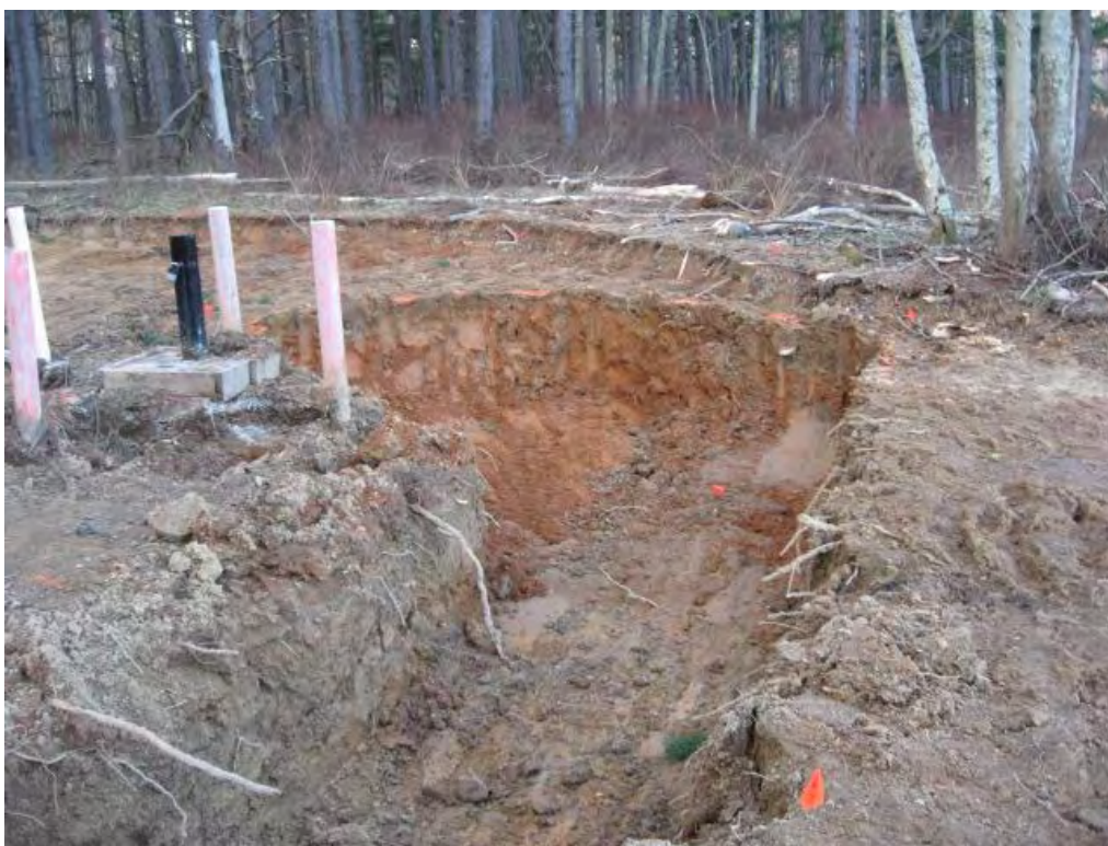
Photo 6 – Central portion of site where target excavation depth was 4-ft bgs.
