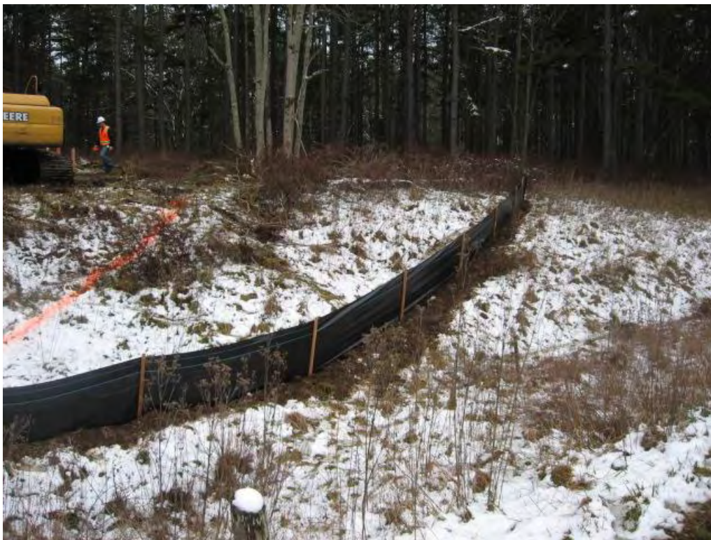
Photo 1 – Silt Fence installed in northwest portion of the work area prior to excavation.
