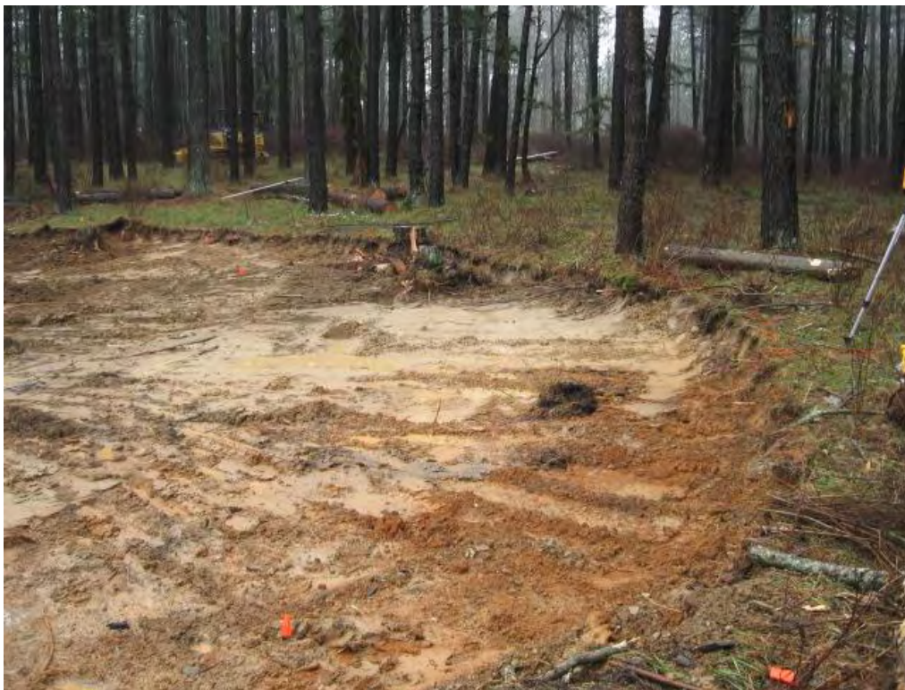
Photo 5 – Southern portion of excavation footprint after target depth of 1-ft bgs achieved.
