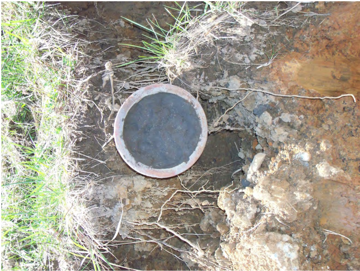
Photo 10 - View to the South of plugged Terra-cotta pipe.
