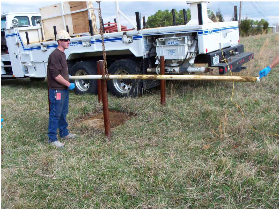
Photo 2 - View to the North West of abandonment of well 57-MW1.
