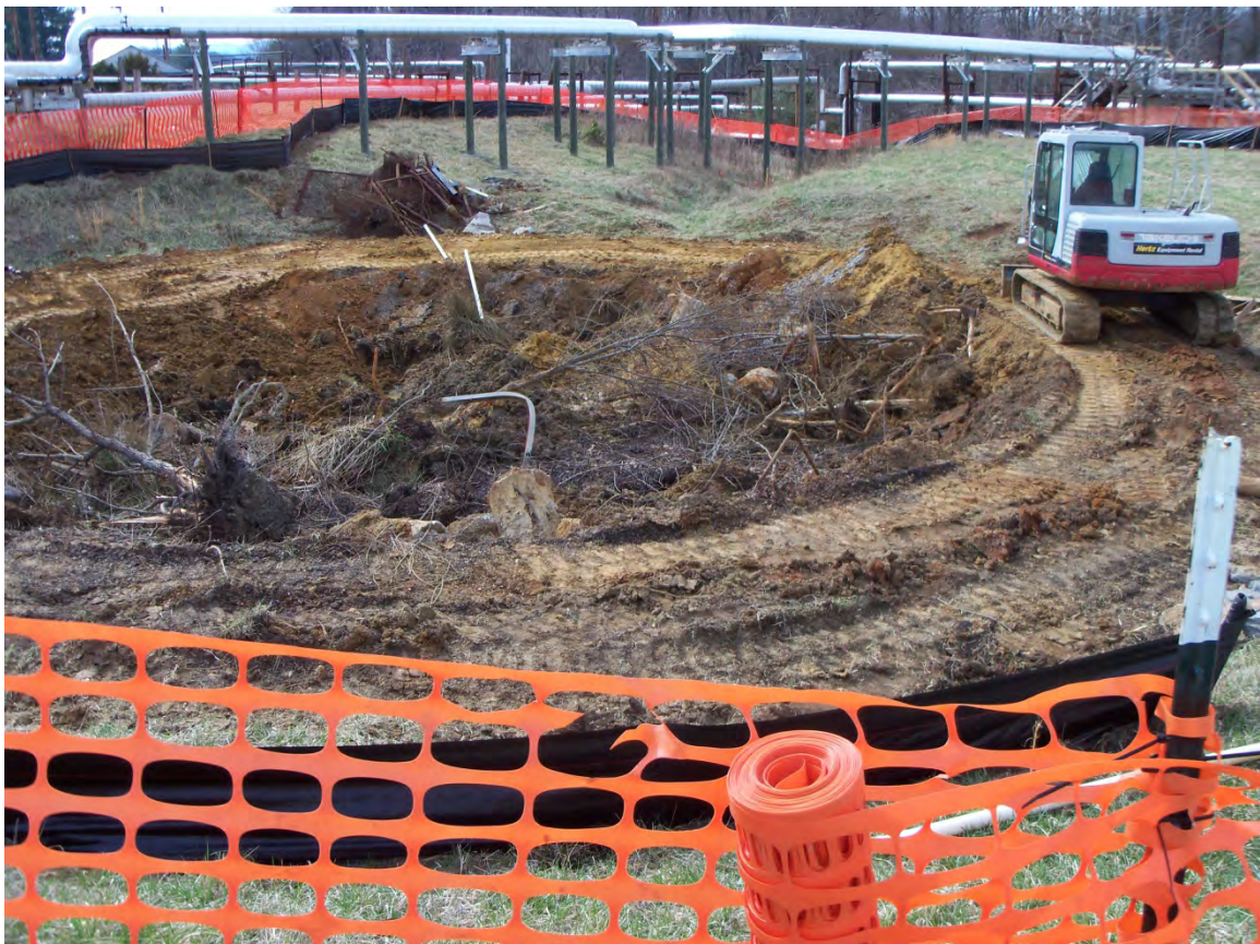
Photo 4 - View to West of silt fence installation, barrier fence, and separation of fencing from the pond.
