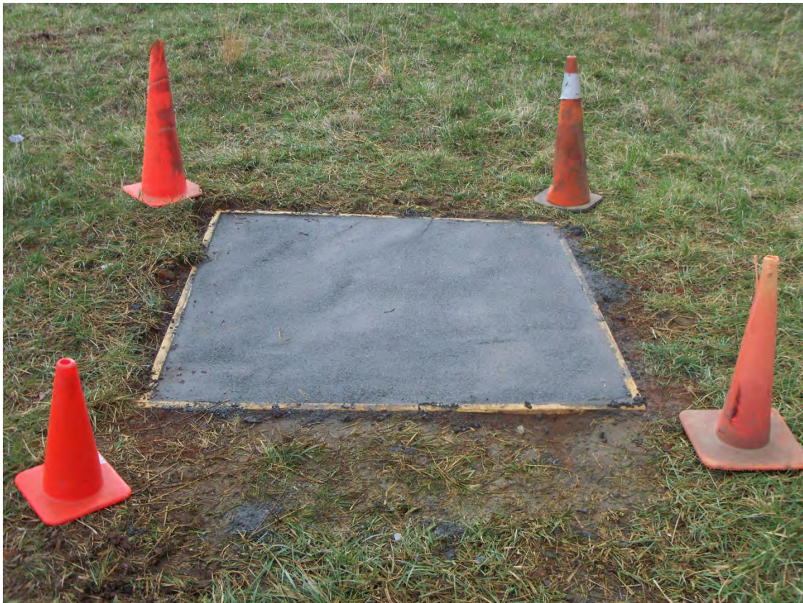
Photo 3 - Completion of abandonment of 57 MW-1.
