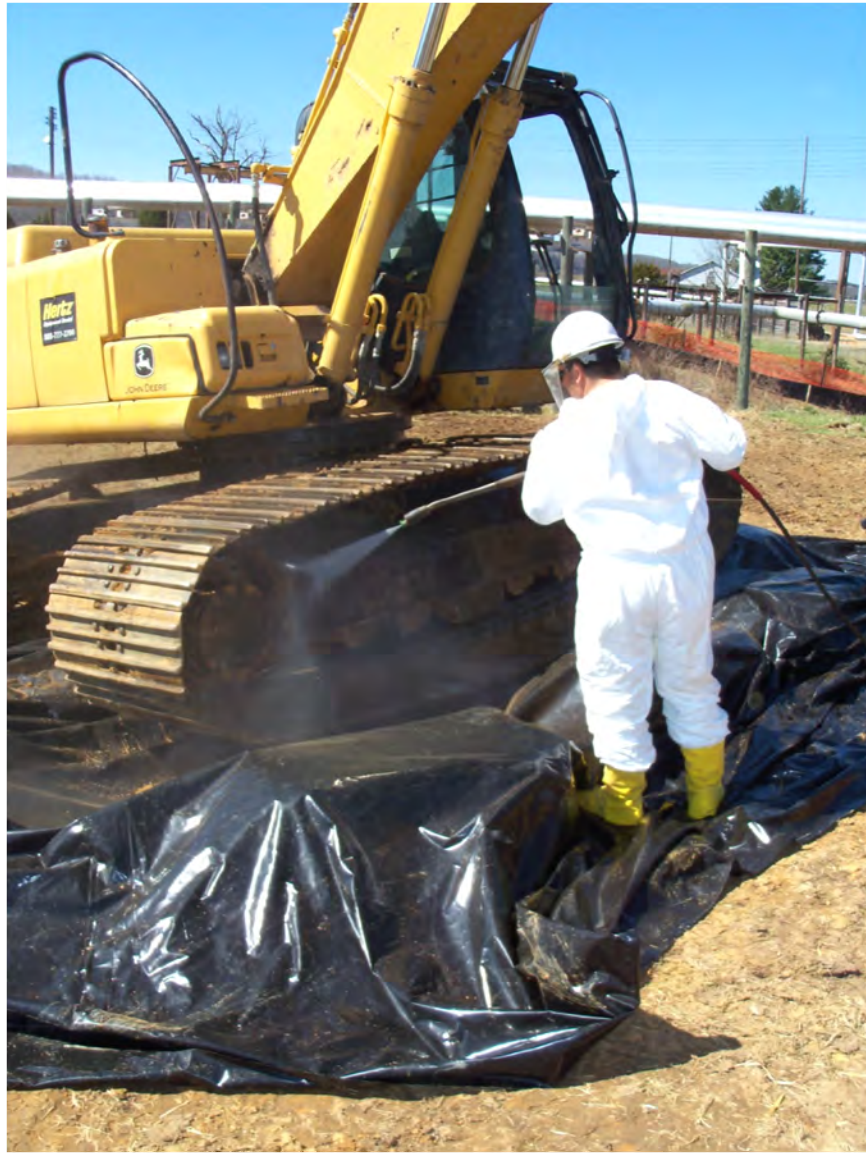
Photo 9 - View to the South of decontamination procedures.
