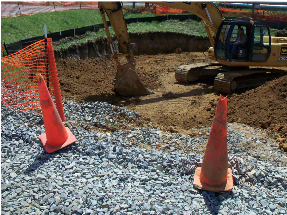
Photo 11 - View to South East of clean backfill and compaction.
