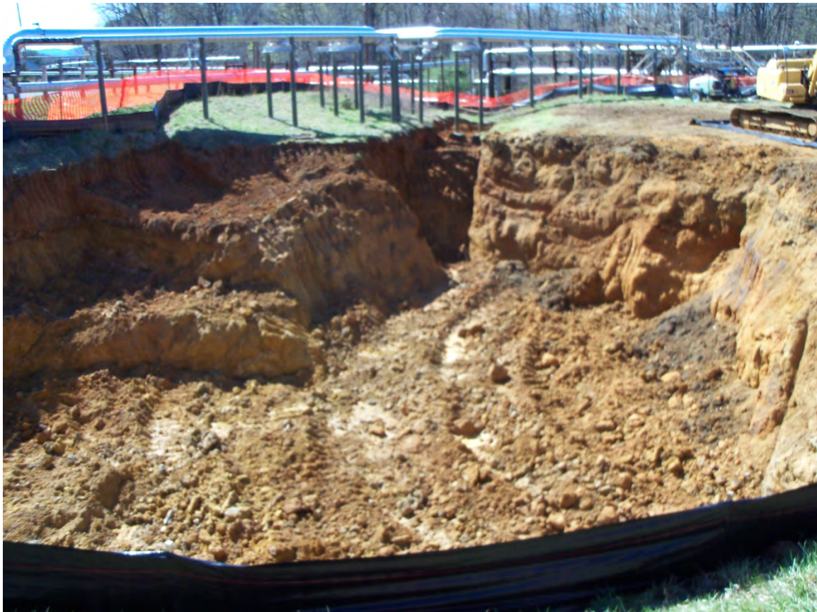
Photo 8 - View to the West of removal completion of contaminated soils.
