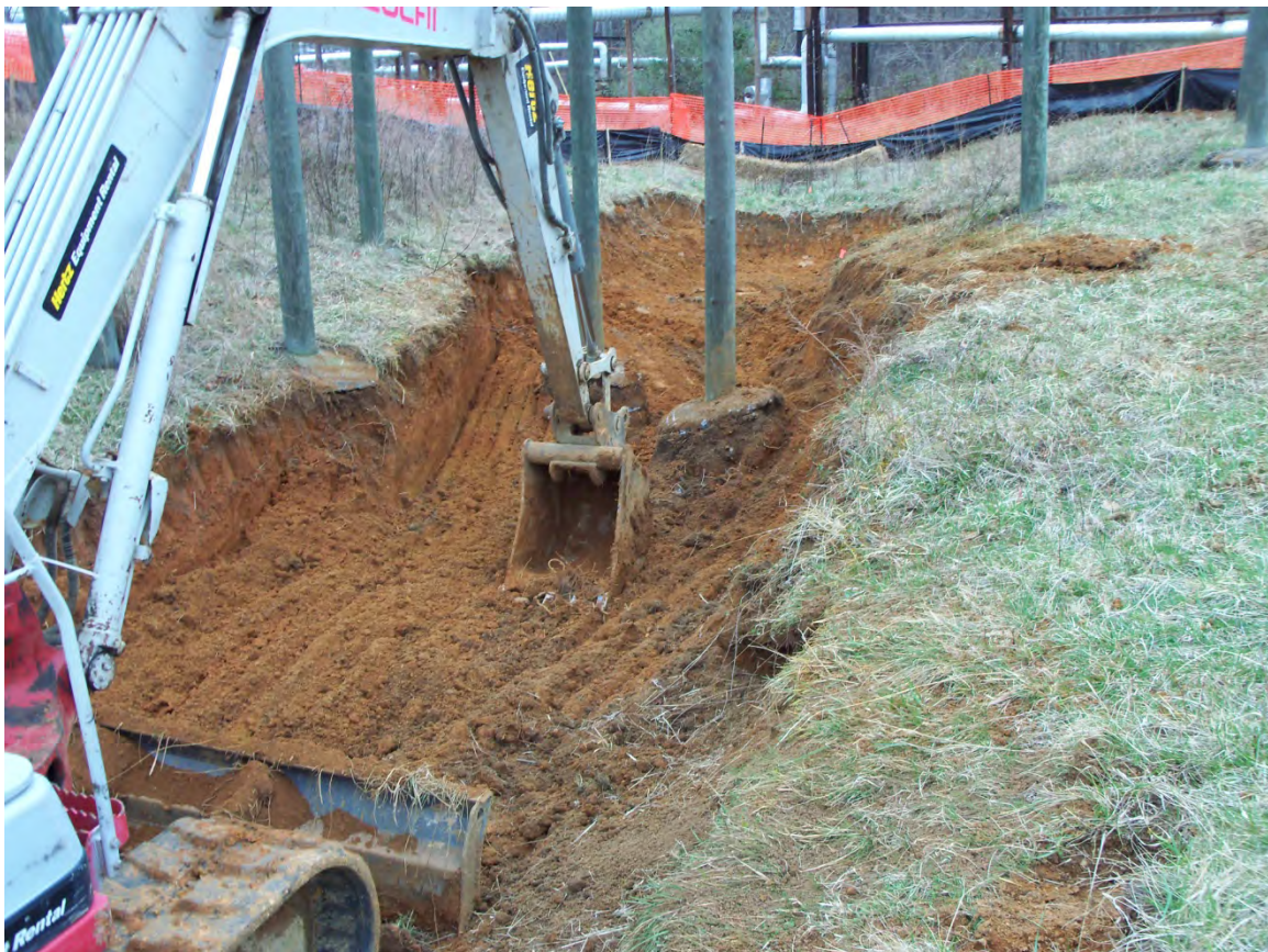
Photo 6 - View to the West of the excavation around steam line supports.
