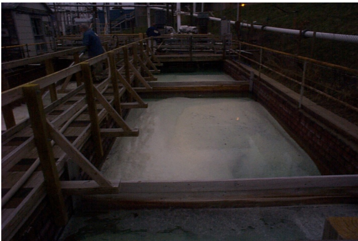
Photo 2. SSA 63 – Nitrocellulose C-Line Boiling Tub House Settling Pits (Bldg 3020).
