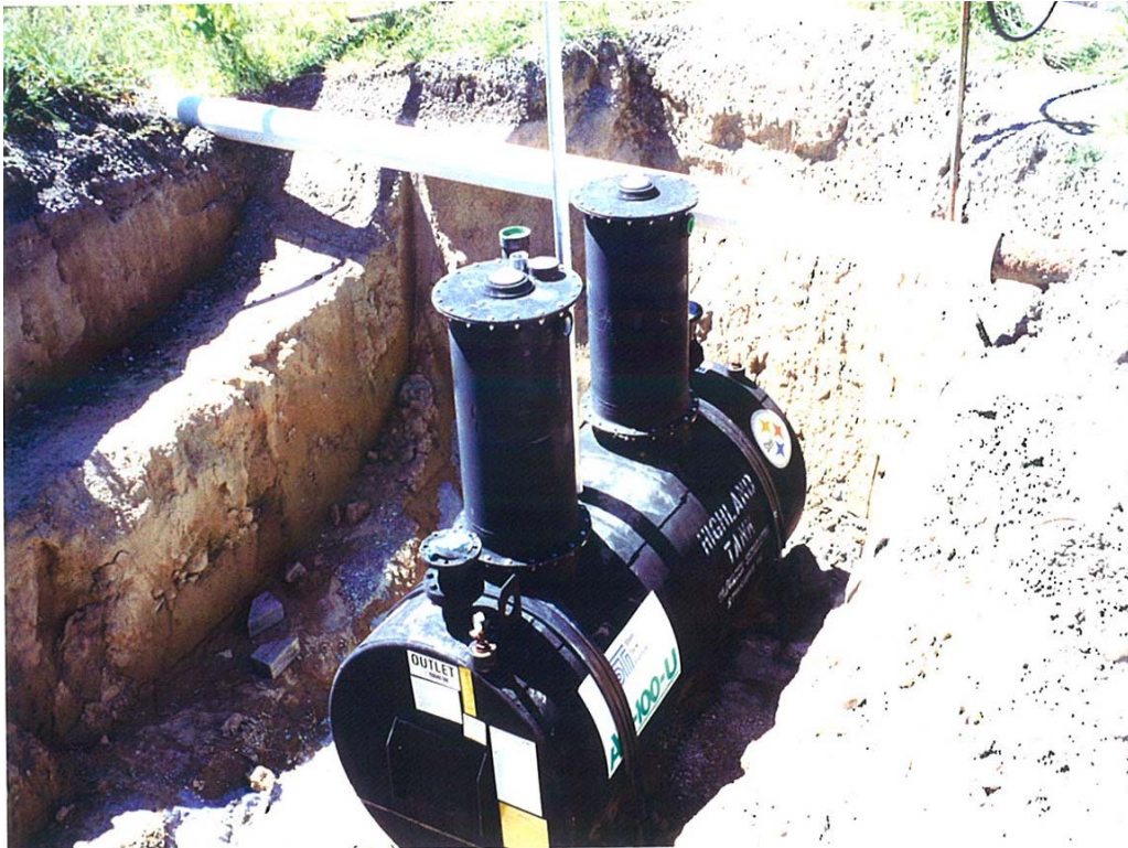
Photo 1. SSA 70 – Installation of 550-gallon oil water separator in 1999.
