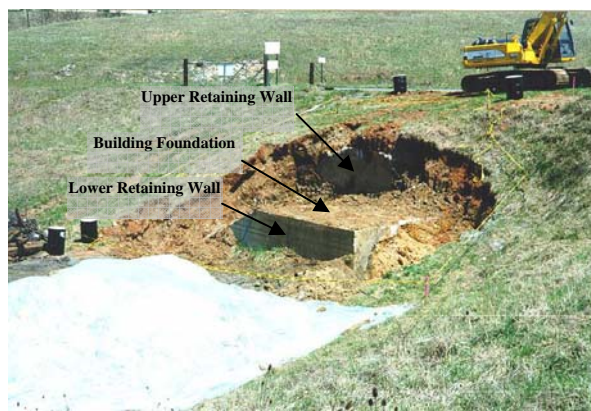
Exposed building foundation attached to lower retaining wall (northeast view)
