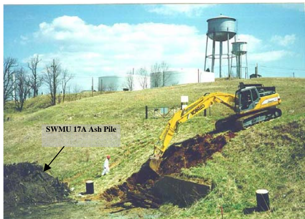
Preliminary soil and debris removal north of the retaining wall (northeast view).
