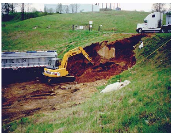
Soil removal from beneath and surrounding the foundation (northeast view).
