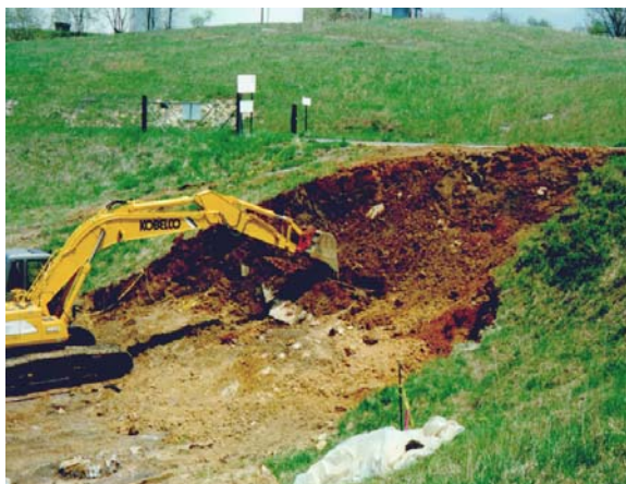
Destruction and removal of upper retaining wall. (northeast view)
