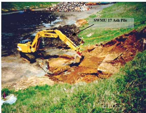
Foundation destruction and removal (northwest view)
