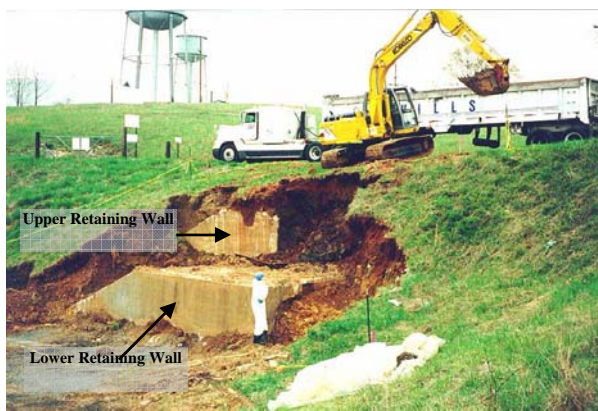
View of concrete retaining walls during soil removal activities (northeast view)
