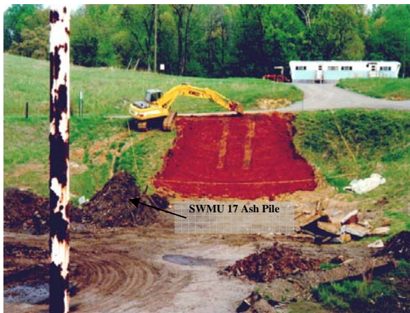
Clean soil backfill and grading activities (east view)
