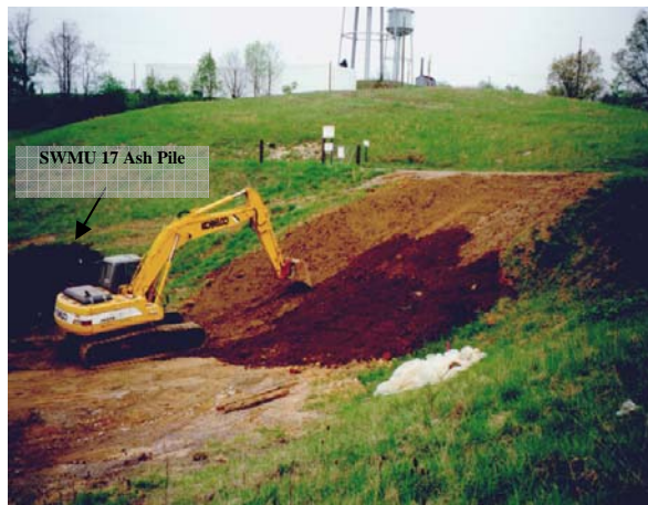
Topsoil backfill and grading activities (northeast view).
