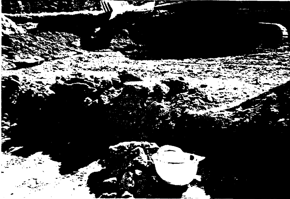
Photograph 7: Continued excavation of approximately 18 inches of soil from the ISP.
