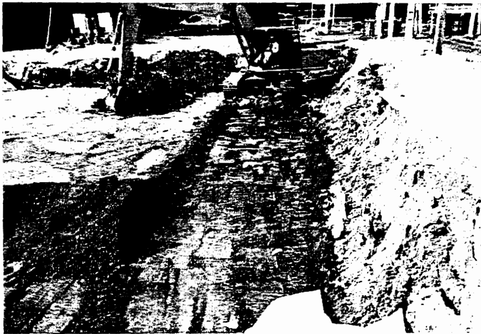
Photograph 6: Additional excavation of approximately 18 inches of soil from the bottom of the original ISP excavation.
