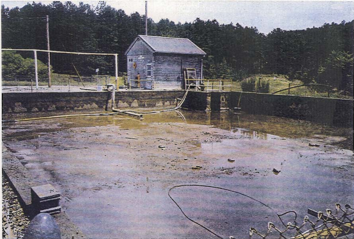
Photograph 1: Incinerator Spray Pond (ISP) with metal piping removed.
