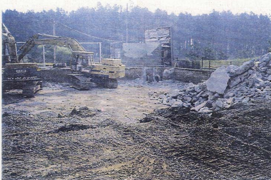
Photograph 3: Concrete removal from the ISP.
