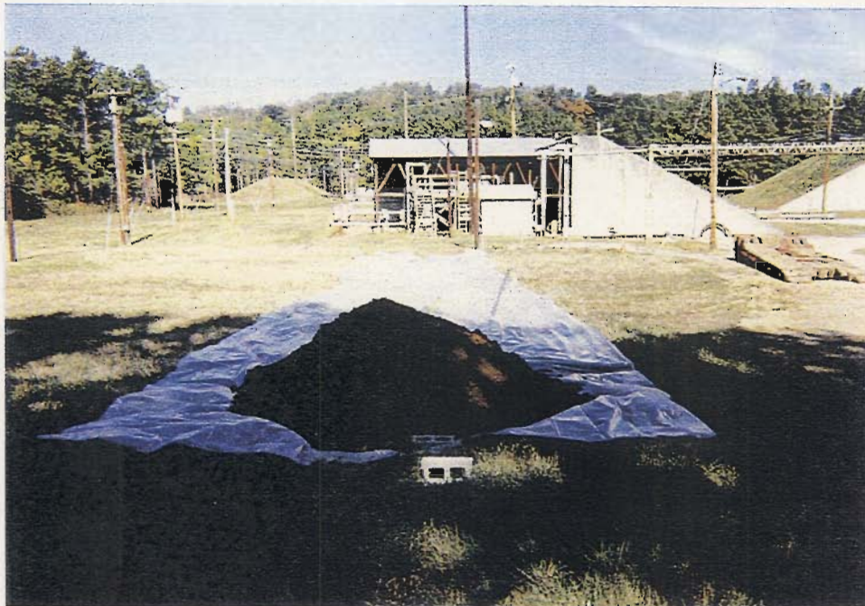
Photograph 9: Staging excavated material on plastic.
