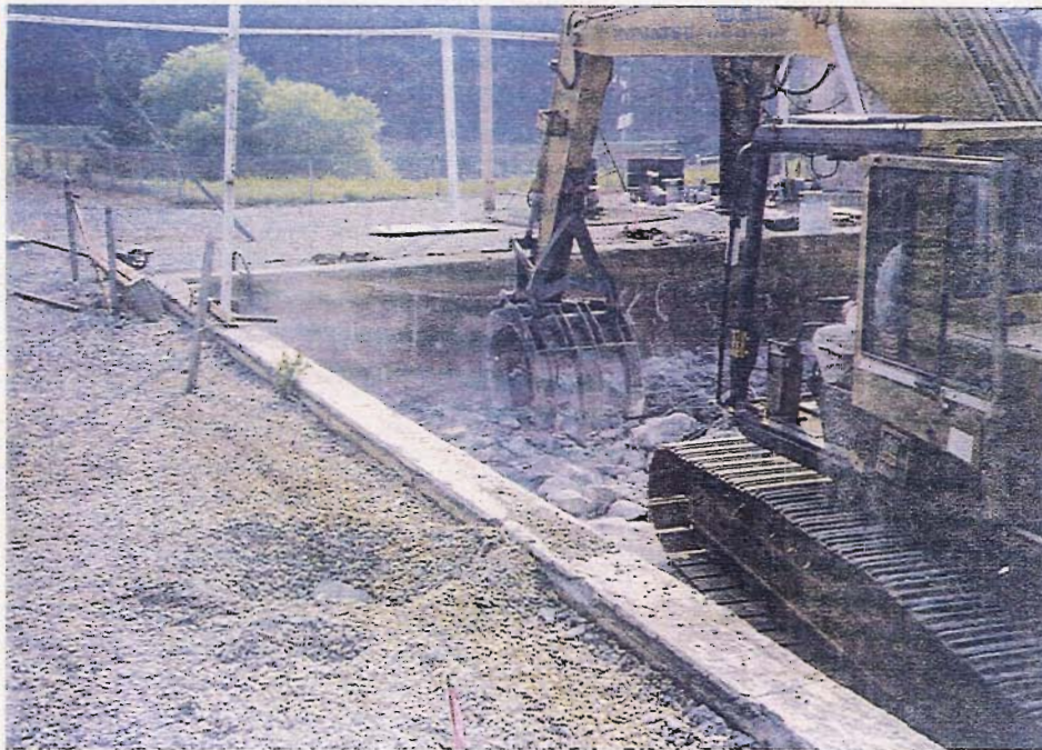
Photograph 2: Removal of the concrete base of the ISP.
