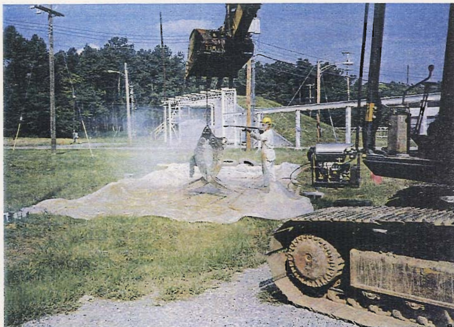
Photograph 5: Decontamination of excavation equipment.
