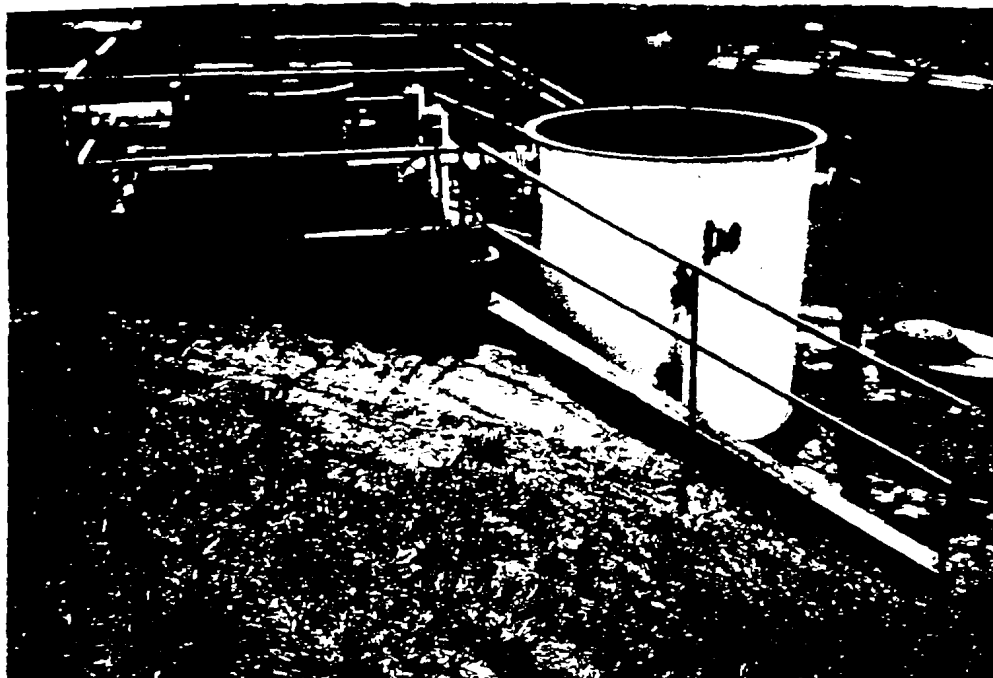
11f. Overview of the Nitroglycerin 1 Neutralization Tank (far right). Note the tank to the left of the unit is the concentrated sulfuric acid feed tank.
