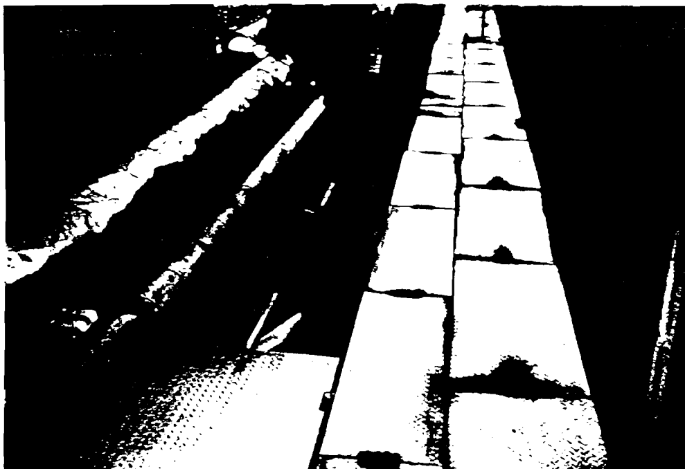
2b. Stainless Steel Flume and Concrete Secondary Containment Gutter (left).
