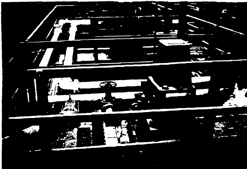
19a(ii). Influent pipes and Equalization Basin for A-B Line Acidic Wastewater Treatment Plant.
