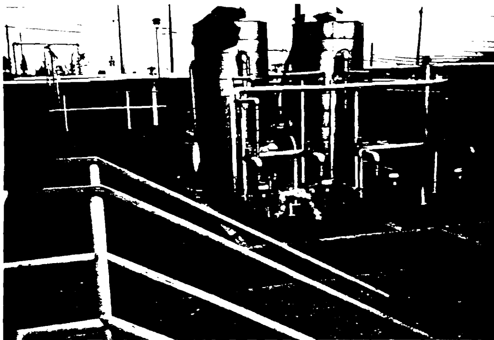
2c(ii) Sump for Equalization Basin overflow.
