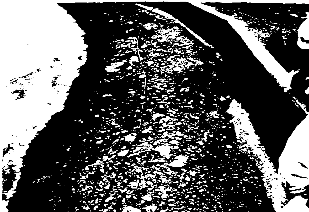
10a(iii). Soil/cement/clay liner for equalization basin for Biological Treatment Plant. Note cracks and discontinuity in liner (center).
