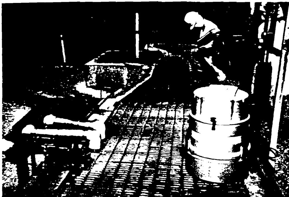
10k. Effluent Flume and sampling station for the Biological Treatment Plant.
