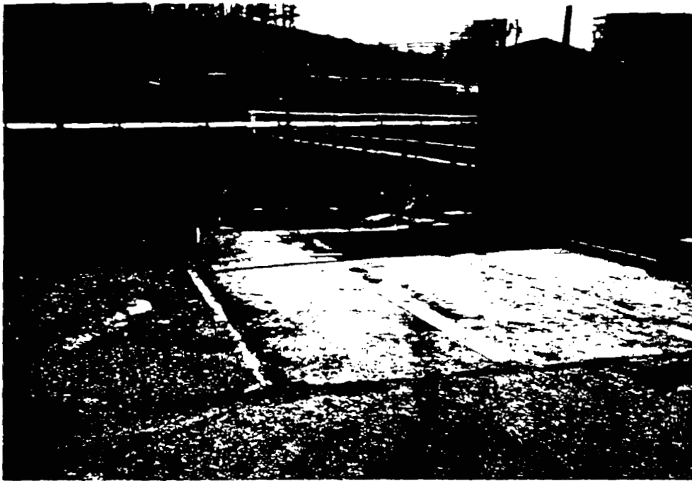
70(i). Heavy Equipment Maintenance Shop Steam Cleaning Area. Note the cracked curbing. Sump in the lower background of the pad discharges to the oil-water separator.
