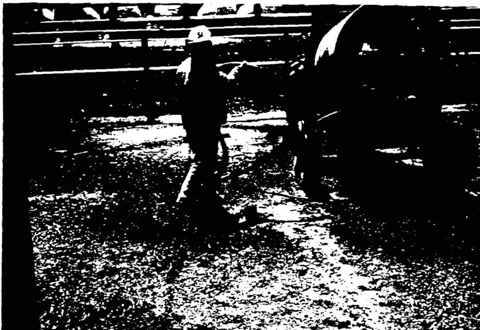
75(ii). Waste oil underground storage tank (A-421). Operator removing hose from inlet. Note oil stains and spillage on ground.
