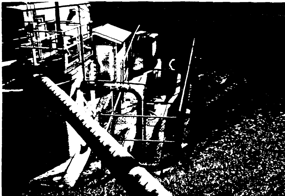
3i. View of the Final Neutralization Tank (left). Note the Parshall Flume to the right of the tank.
