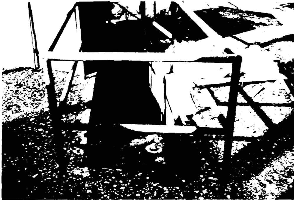
20e. Parshall Flume from Acid-Brick-Lined Effluent Sump (20c) of C-Line Acidic Wastewater Treatment Plant. Note stains and broken Lime Bag.
