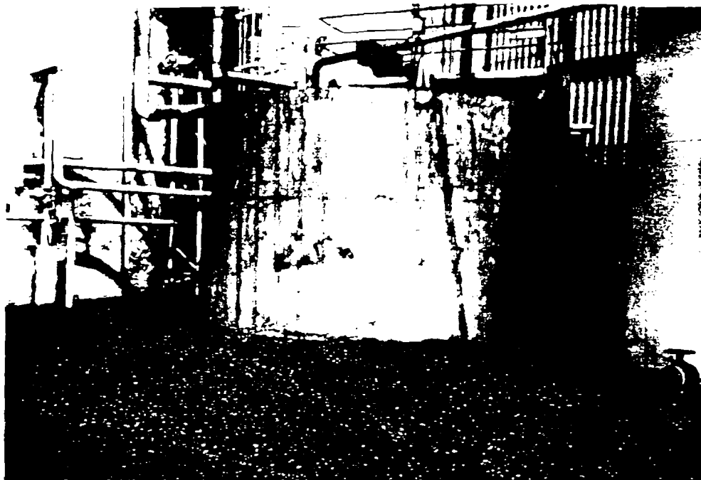
10h. Sludge Thickener Tank (center) adjacent to the Biological Treatment Plant.
