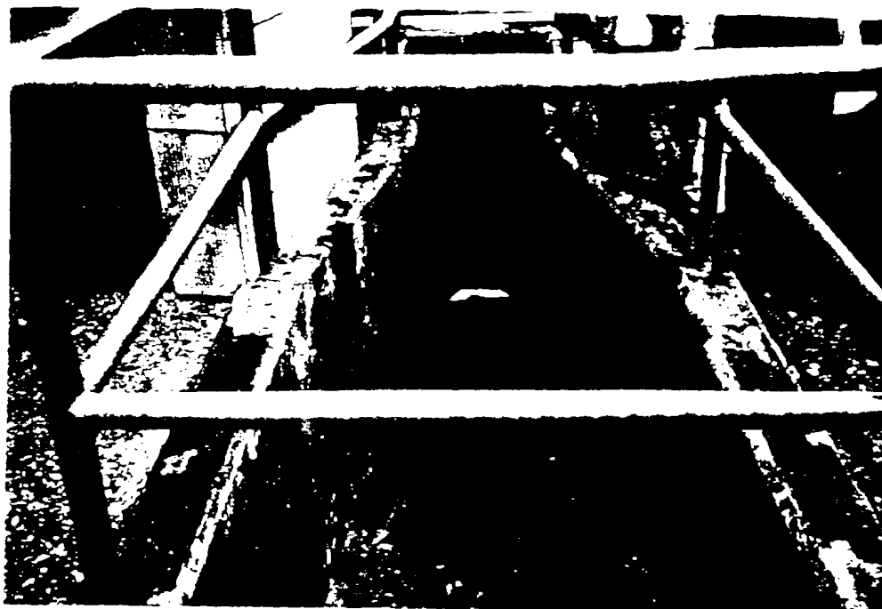
19g. Parshall Flume for A-B Line Acidic Wastewater Treatment Plant.
