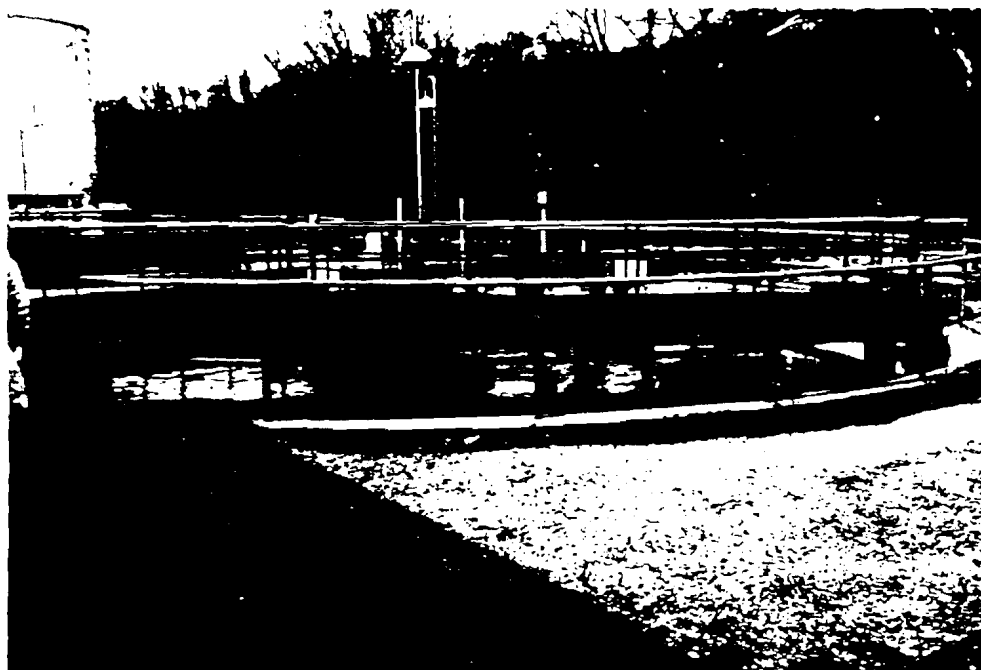
10f(i). First Weir Clarifier for Biological Treatment Plant.
